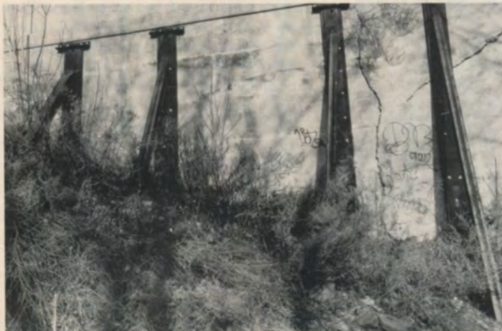
The ravages of time: in 1951, an inspector in Naperville, Illinois, noted the durability of different cements (below). Steel beams reinforce a bridge in Brooklyn (left), where repair funds have been cut.
