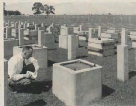
The ravages of time: in 1951, an inspector in Naperville, Illinois, noted the durability of different cements (below). Steel beams reinforce a bridge in Brooklyn (left), where repair funds have been cut.
